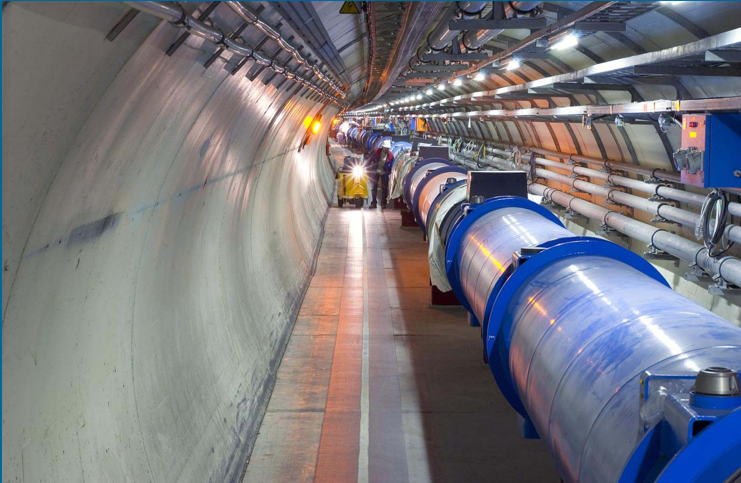
CERN-LHC: part of the 27 km tunnel
